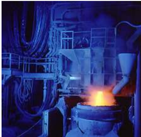
Electric Arc Furnace (EAF)
